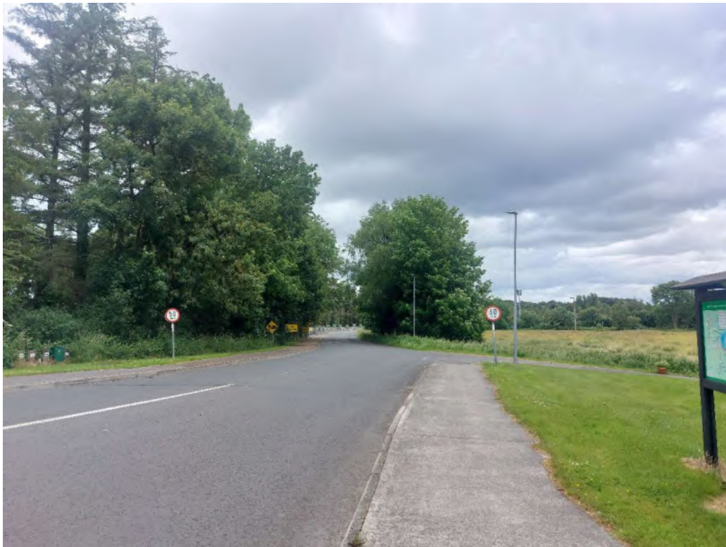
Plate 12-23: View of south-west end of L2020 (CH010), facing north.
