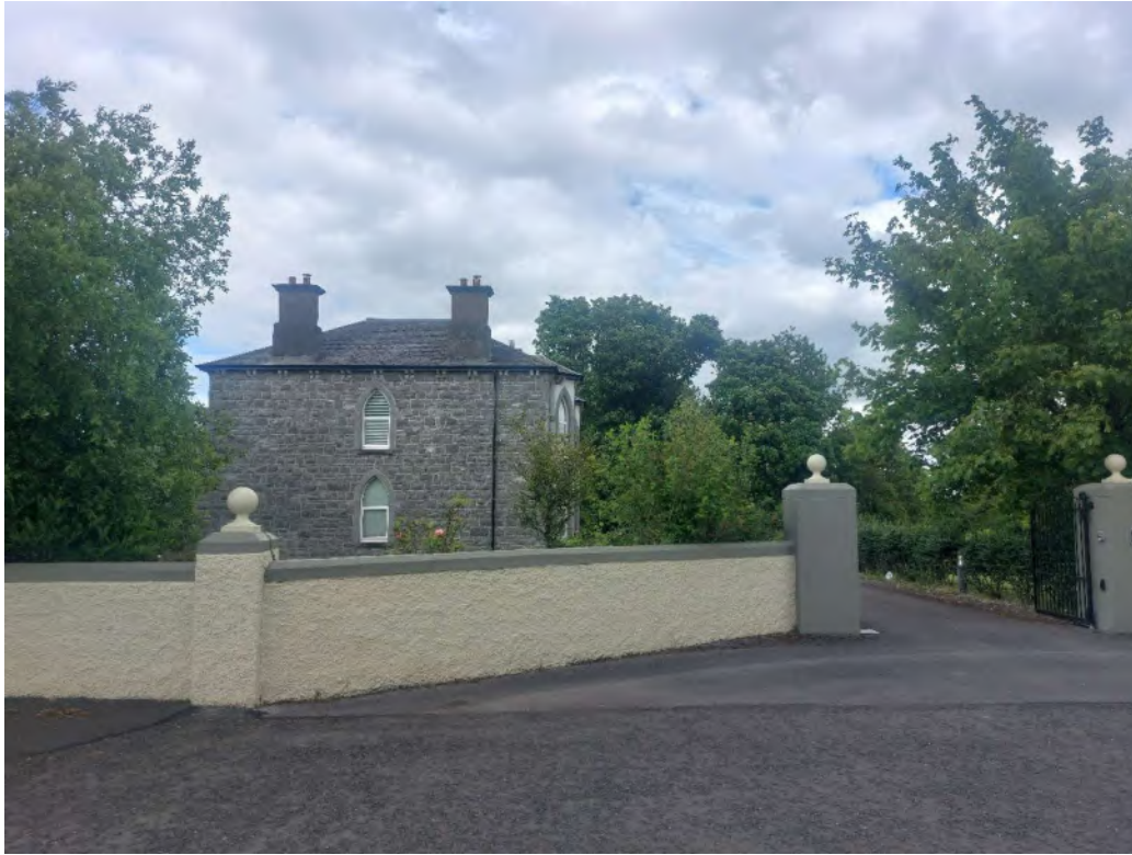
Plate 12-24: View of CH1005 (Presbytery), facing north-east.
