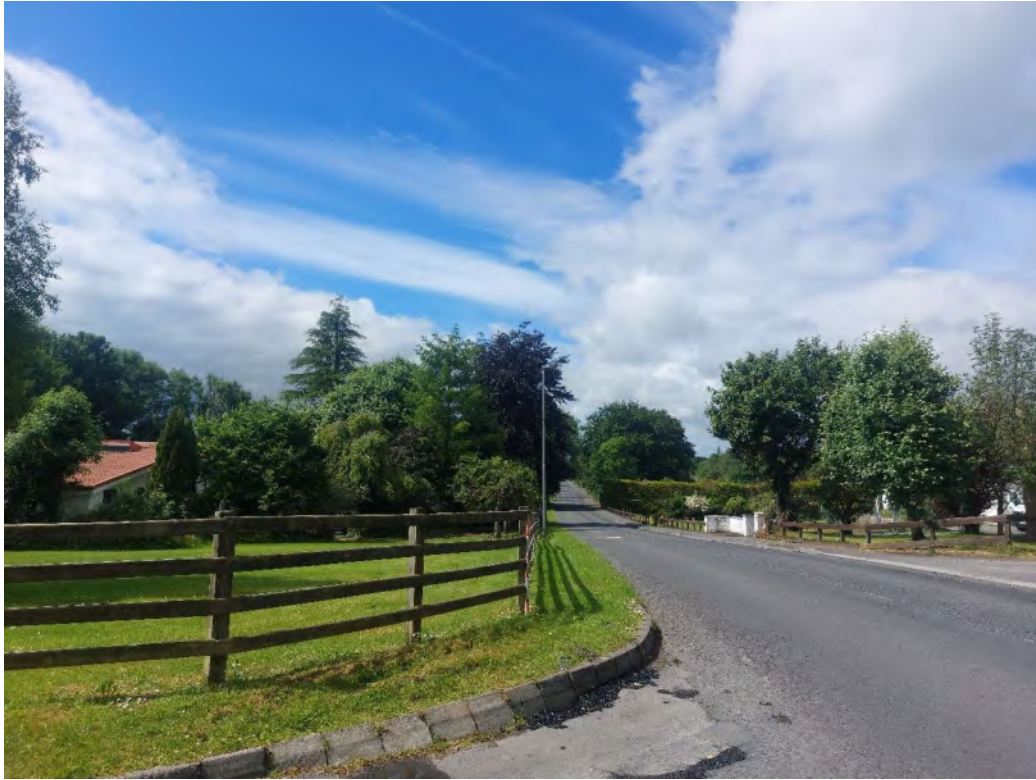
Plate 12-20: View of former location of CH009 (vernacular structure), facing south-west.
